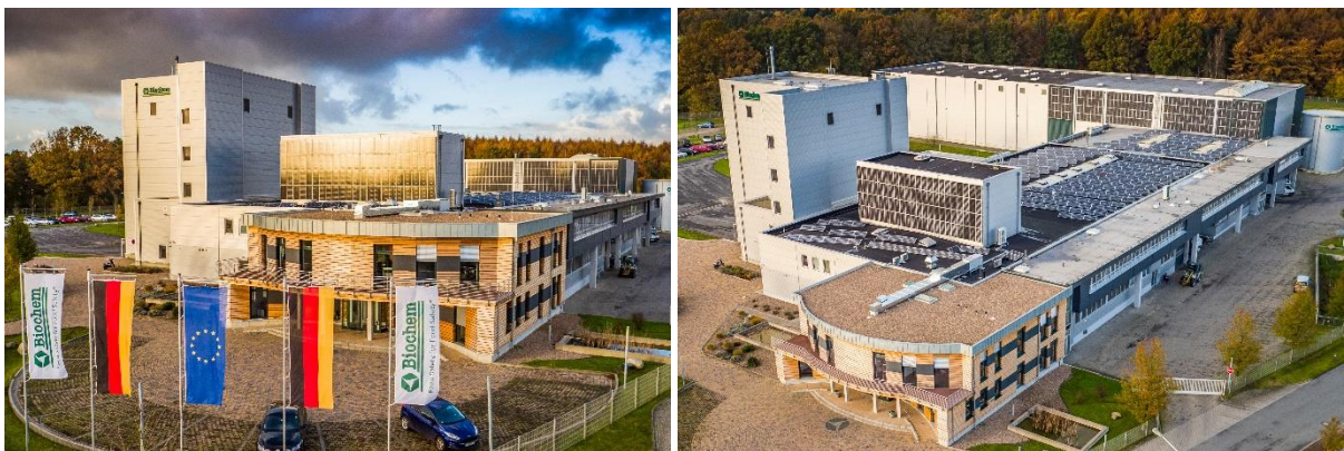
Biochem production facilities (Lohne, Germany)
